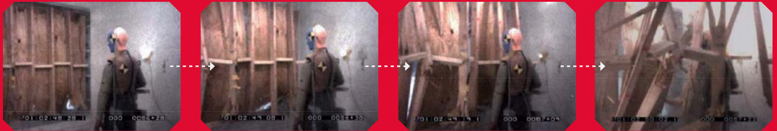
Failure of wood building/trailer at 1.5 PSI
